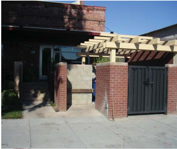
Screening of outdoor trash containers
