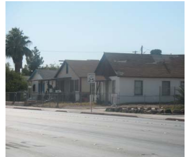
Up until the present, residential development has primarily comprised low density, almost exclusively single-family dwellings.
