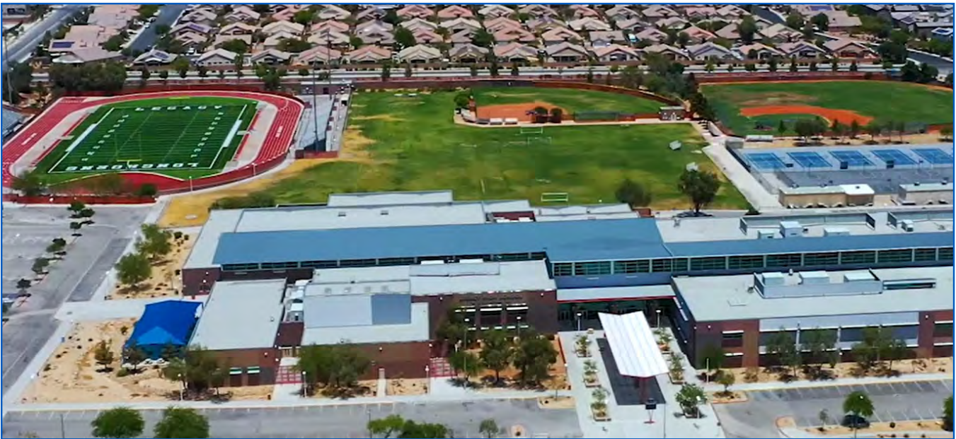
Legacy High School, Clark County School District
