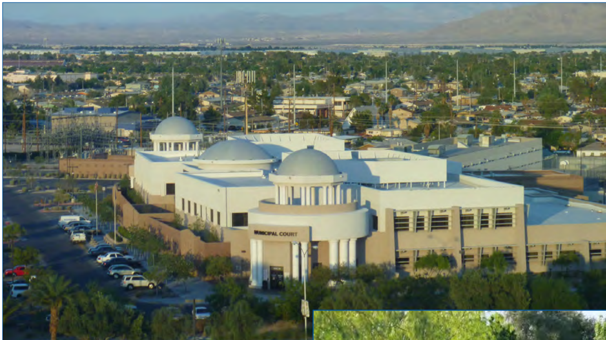
North Las Vegas Municipal Court and Justice Facility
