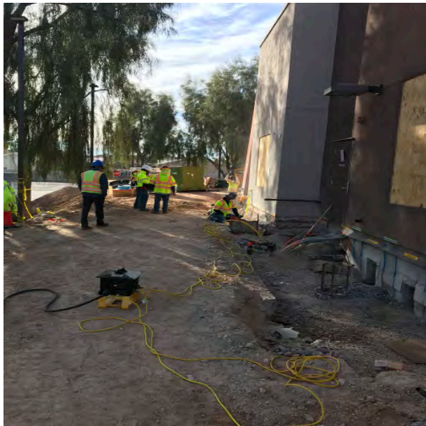
Fire Station 52 Remodel
