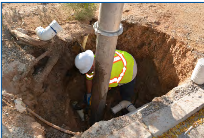
6" Water Main Repair using the safe dig.
