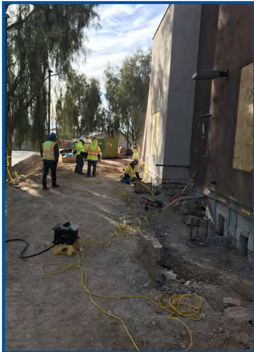
Fire Station 52 Remodel
