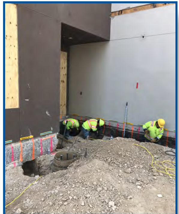
Fire Station 52 Remodel
