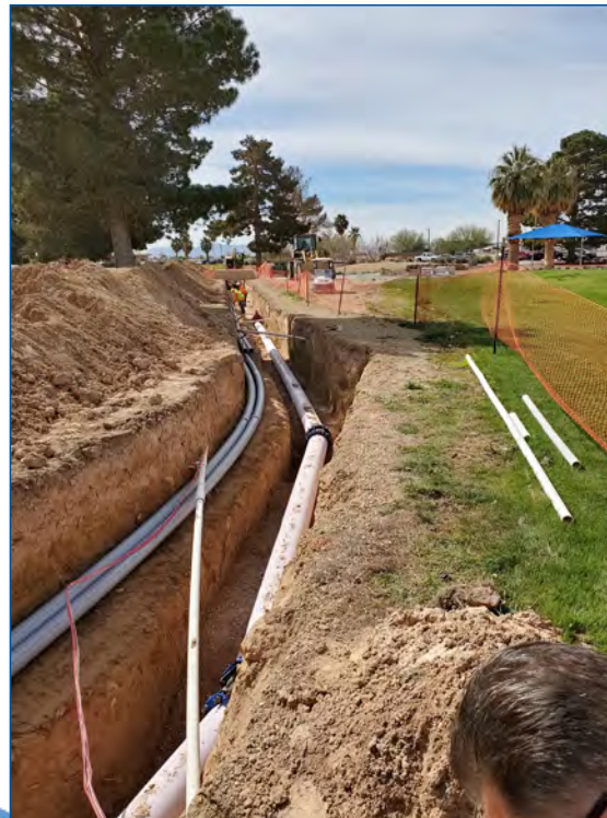
Nellis reuse water line install
