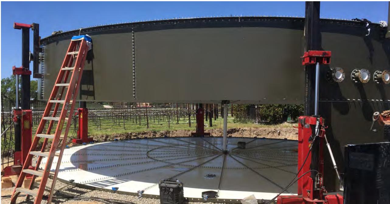
Example of Bolted Tank Construction
